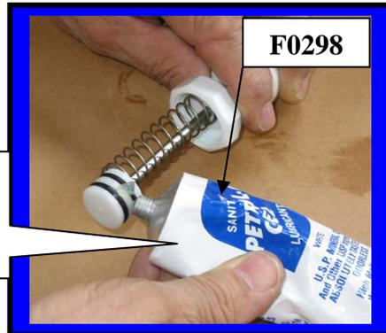
Installing **Plunger Assembly** into Faucet body
